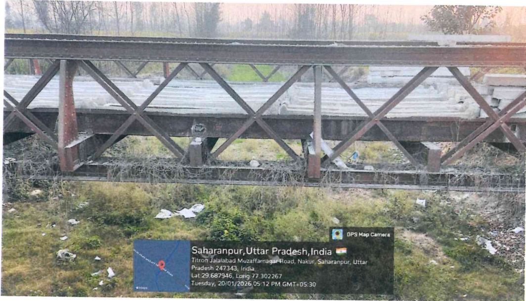
Location 2: Titron Jalalabad Muzaffarnagar Road, Nakur, Saharanpur (Bridge Location)
