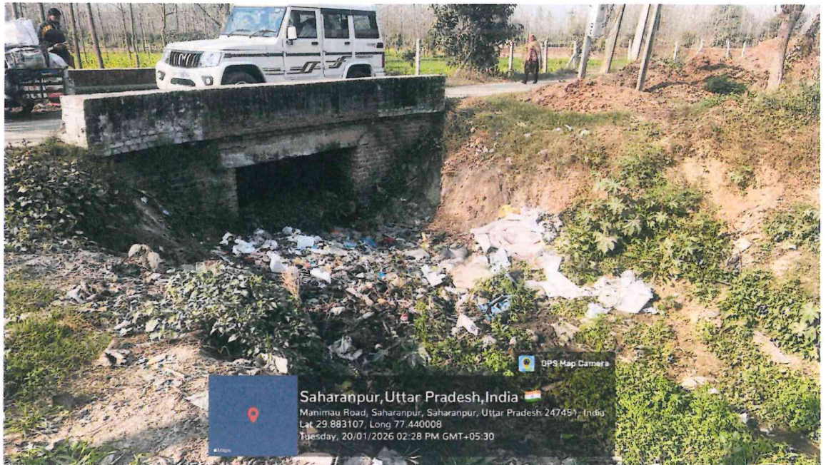
Location 7: Drain at Manimau Road, Saharanpur
